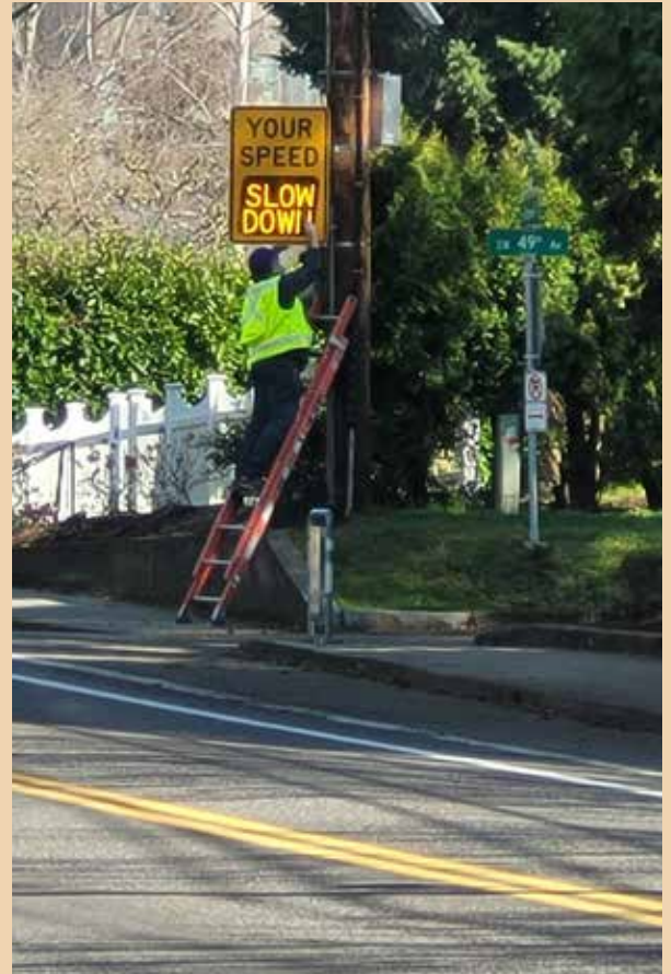
Portland transportation employee installs a speed-reader sign in the Hayhurst neighborhood at SW 50th and Vermont.
