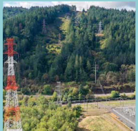
Undated aerial photo of part of PGE's transmission system on the northern edge of Forest Park.
